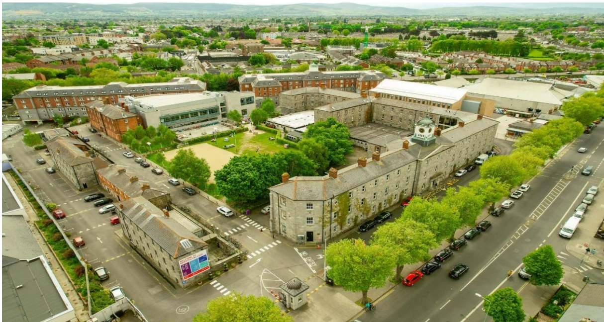
Griffith College South Circular Road Campus, 2024
