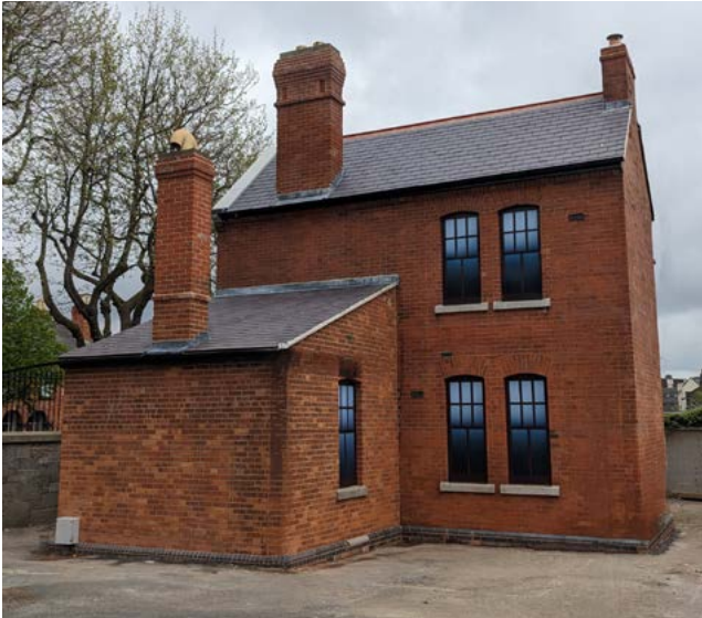
Post-restoration images of the historic Quarter Master House, South Circular Road campus, May 2024.
