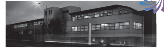
Implementation of the Shared Services Payroll Project where payroll, subsistence and travel expense activities are being migrated to the Education Shared Business Services Centre (ESBS) in Dublin. Organisational restructuring at LWETB Head Office Mullingar, 2019
