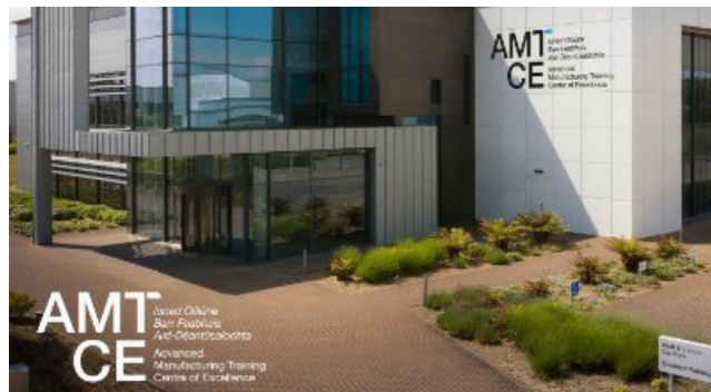
Establishment of Advanced Manufacturing Training Centre of Excellence, LMETB's newest FET facility in 2020
