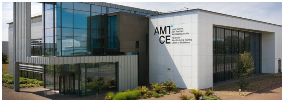
AMTCE building in Xerox Technology Park, Dundalk
