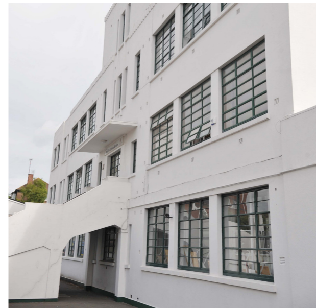
FET Centre, King Street Drogheda: New boiler and associated heating system replacement project, as well as the installation of a full electrical rewire of the building in 2020 and 2021 respectively.
