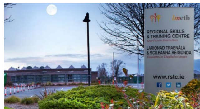
RSTC Dundalk received funding and sanction for a boiler replacement in Summer 2021. In addition, classroom accommodation was repurposed into workshop space to accommodate requirements of enlargement of apprenticeship provision.
